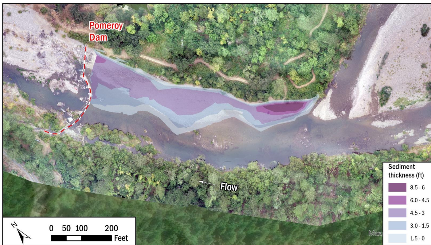
Figure 3-10. High resolution orthoimagery collected August 22, 2024, with estimated thicknesses of the impounded river-right gravel bar. Note bedrock exposures visible in the river-left portion of the channel.
