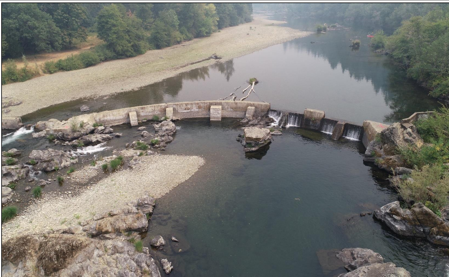
Figure 6-2. Oblique aerial view looking upstream at Pomeroy Dam, river-right bar deposit, and bedrock scour hole downstream of the dam. Photo taken August 22, 2023.
