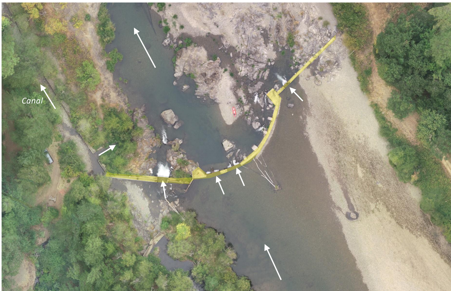
Figure 3-1. Aerial view showing Pomeroy Dam (highlighted in yellow), canal and existing flow paths (white arrows). Photo taken August 22, 2023.
