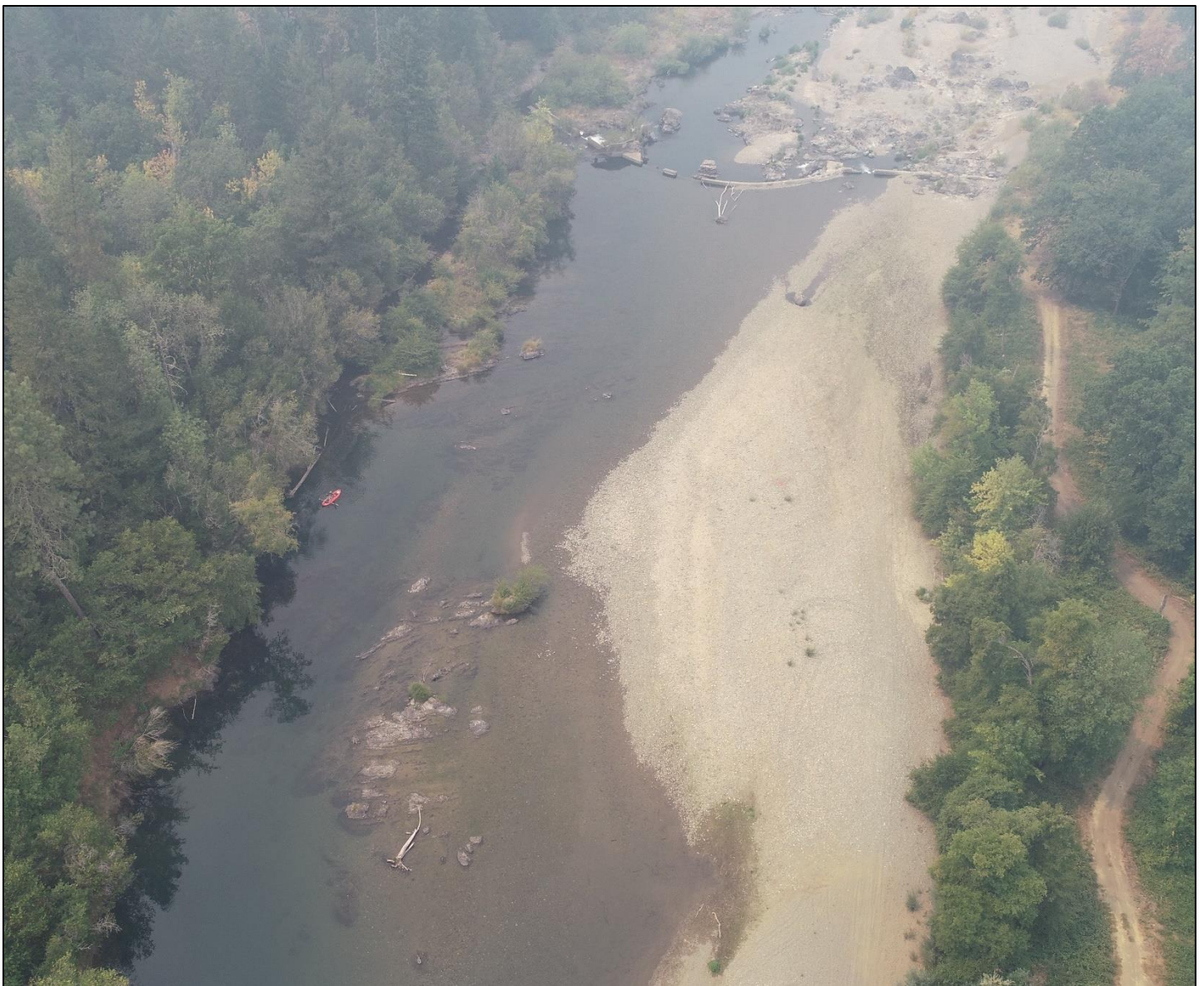
Figure 3-5. Oblique aerial view looking downstream at the lower reservoir and dam. The Galice Formation is visible through the water on the river-left side of the wetted channel upstream of the dam and throughout the channel downstream of the dam. A red inflatable kayak is visible for scale. Photo taken August 22, 2023.
