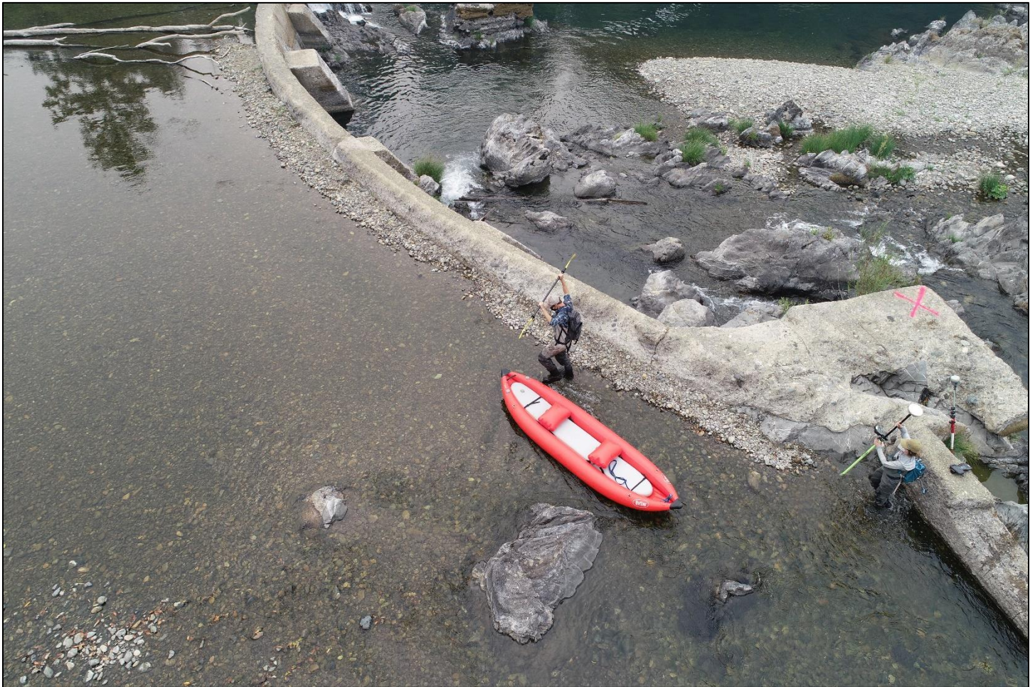
Figure 3-11. Oblique aerial view looking towards river-left of the dam and the gravel-sized sediment impounded behind it. Photo taken August 22, 2023.
